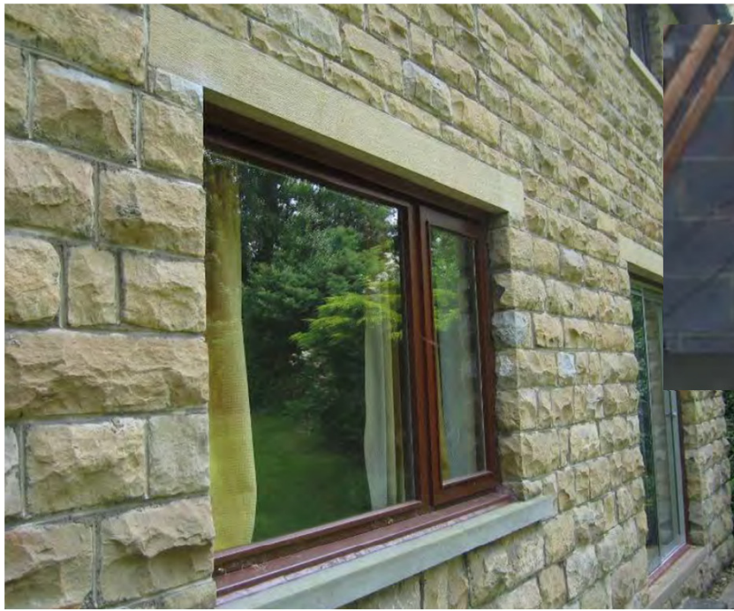
Cavity walls, stone faced with reconstituted stone dressings to openings, concrete block inner skin
