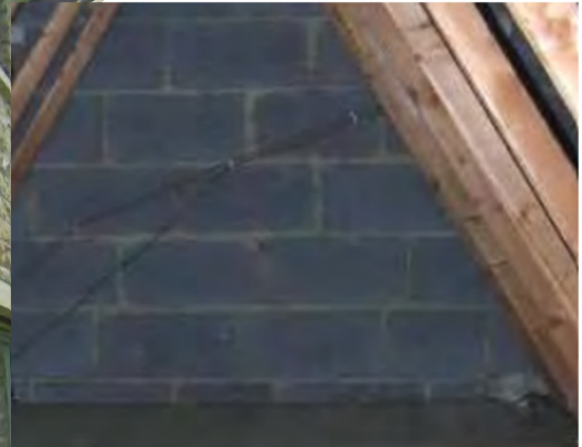
Cavity walls, stone faced with reconstituted stone dressings to openings, concrete block inner skin
