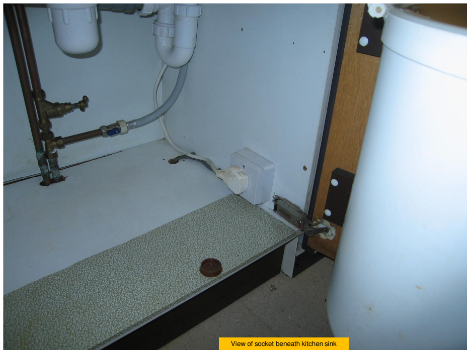
View of socket beneath kitchen sink
