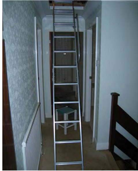
Pre-fabricated trussed rafter roof with fixed ladder to hatch of landing
