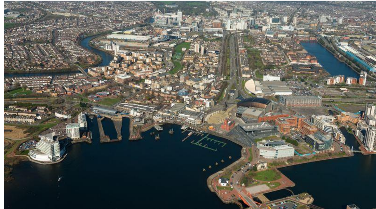
Cardiff Bay Development Corporation regeneration (1,100 hectares of derelict docklands)
